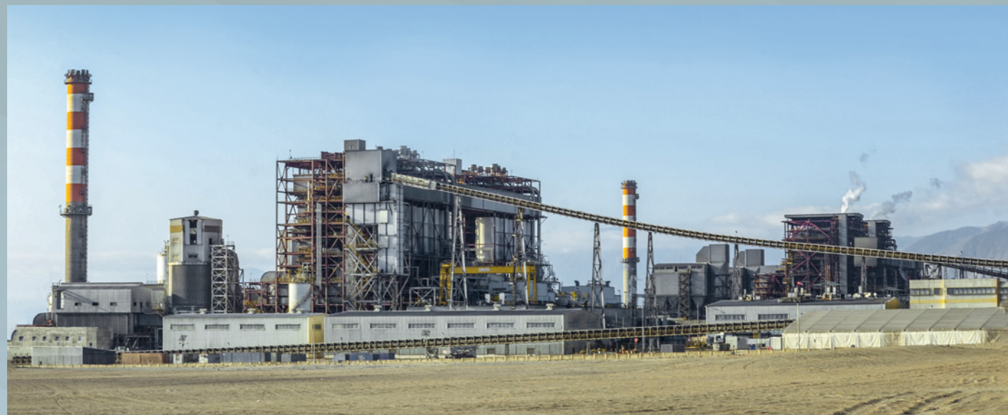
AES coal power plant in Mejillones
