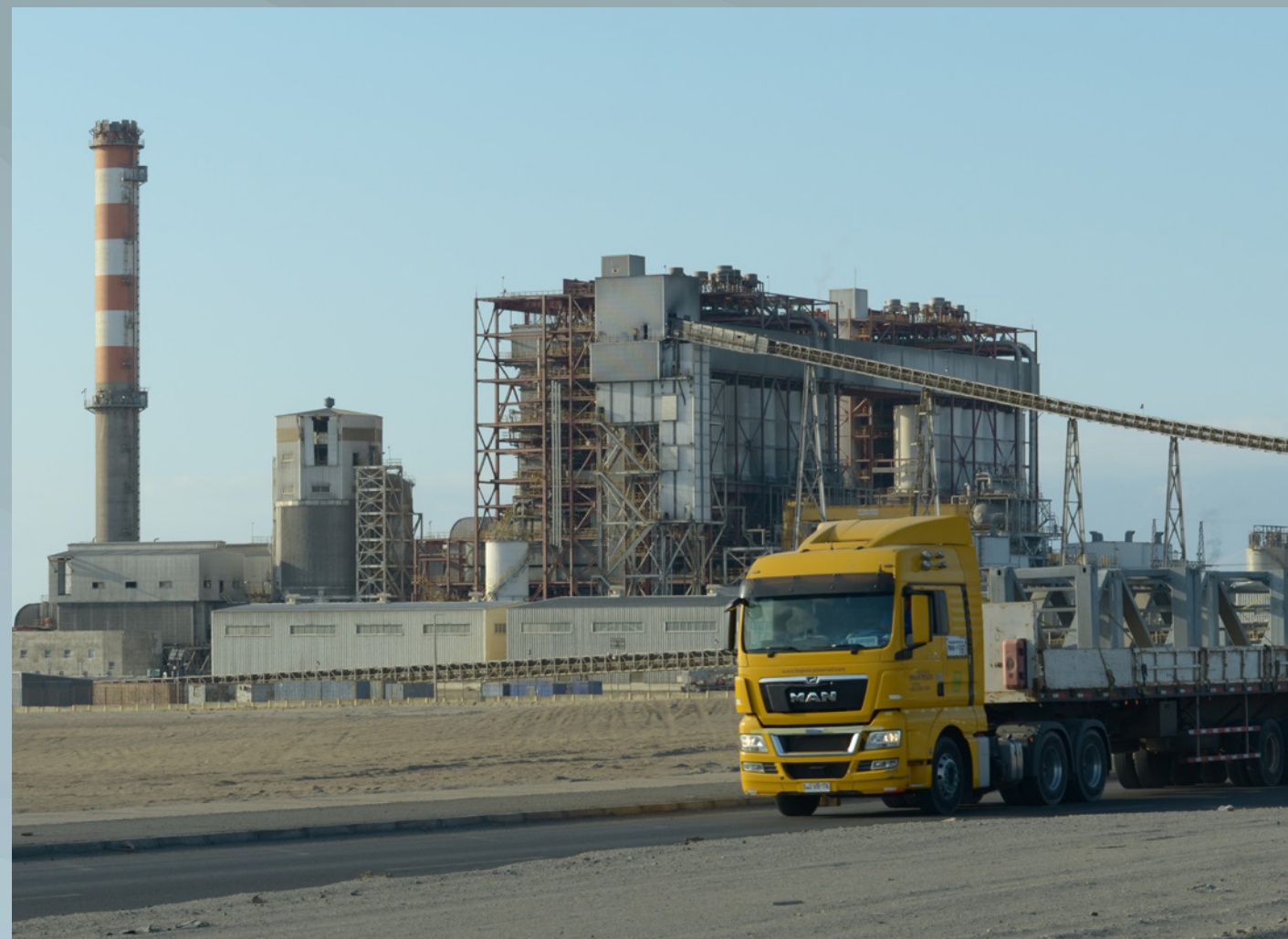
AES coal power plant in Mejillones
