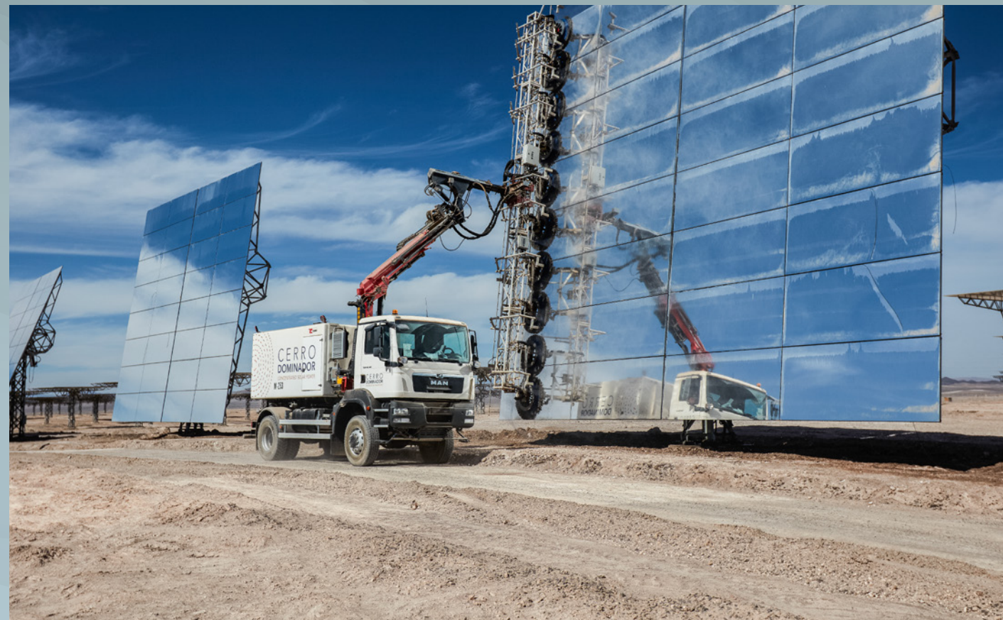
The mirrors of the CSP unit must be cleaned regularly.
