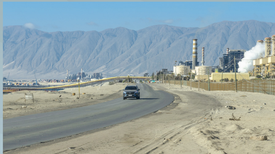
Coal-fired power plants in Mejillone
