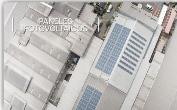
Solar Photovoltaic System in the Food Industry (Puratos)
